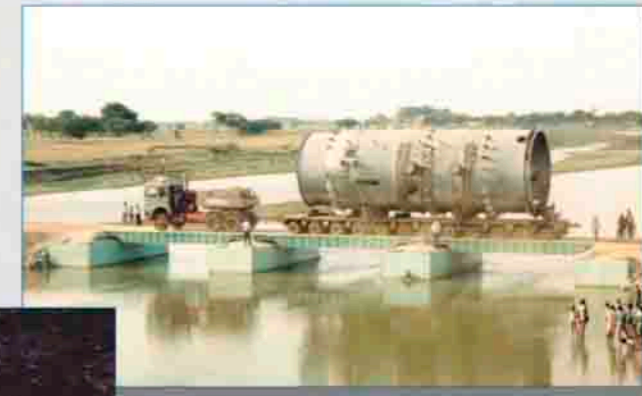
Comprising of Steel pontoons 10m X 3m X 3m & Steel Ramps As Shown In Photographs. Designed / Constructed / Owned By Urmila. Bridge Tested to 410 MT Load.
